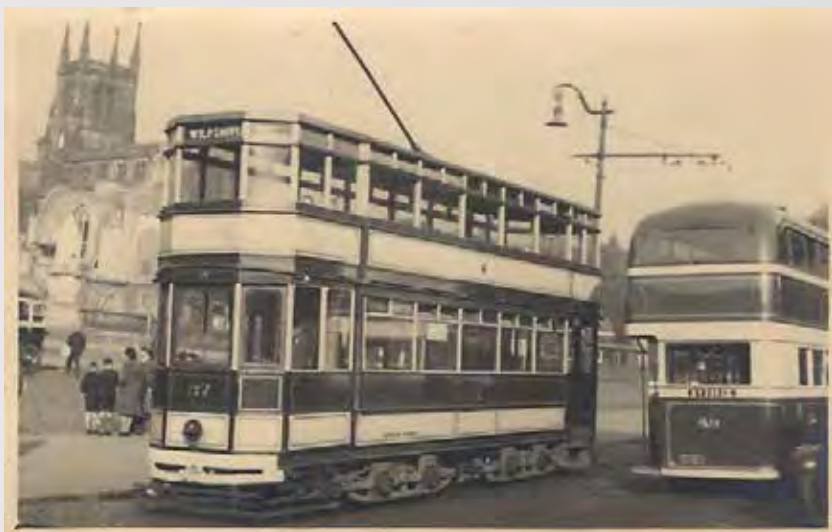
A wartime Blackburn tram
